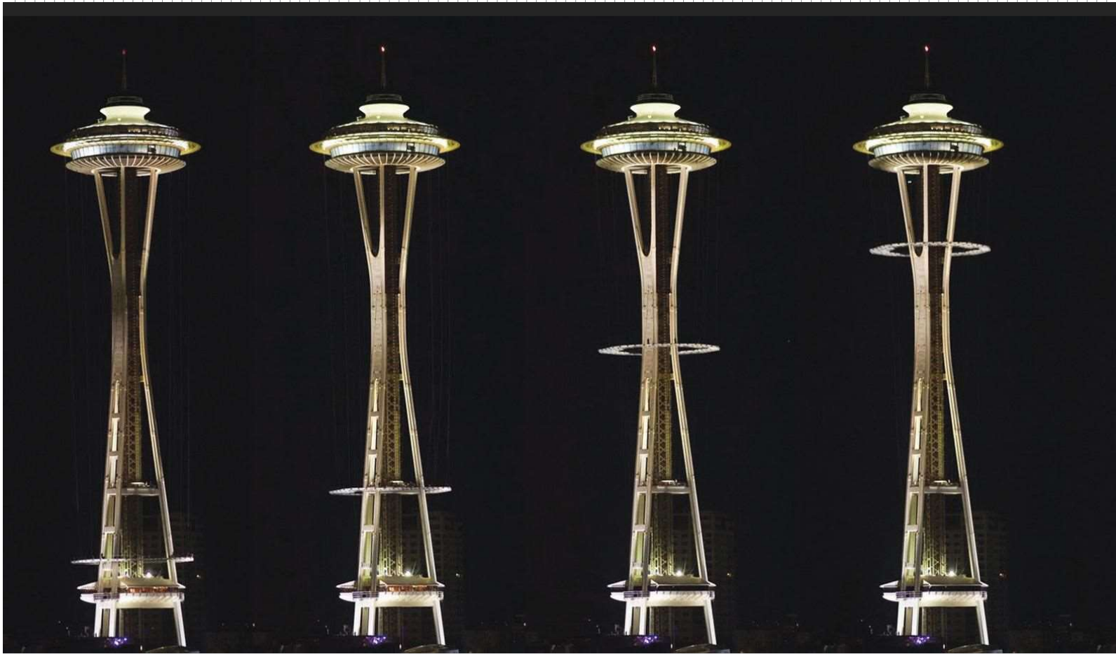
TIME LAPSE The Century Project, Seattle's renovation of the Space Needle, used an elevated platform erected at night and placed 500 ft up.
