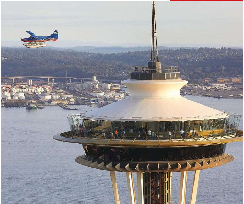
BIRD'S-EYE VIEW The Space Needle renovation adds floor-to-ceiling windows and glass benches to the observation deck.
